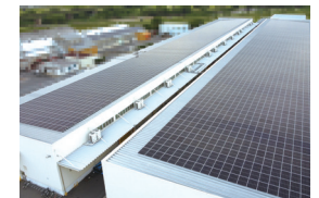
Last year, we started installation of solar panels at the No.10 and No.13 plants
